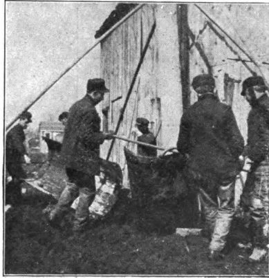
Fig. 13.—Removing Iron Barrel with Bars.
